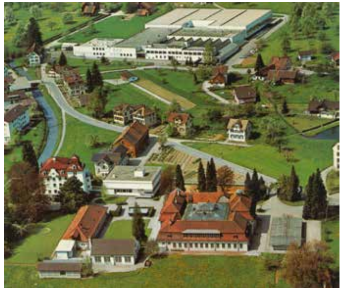
Swiss Silk Bolting Cloth Manufacturing Company of Thal, ca. 1969. Foreground: Former headquarters of Dufour & Co., built in the 19 th century. Background: The factory today. Sefar company archives
