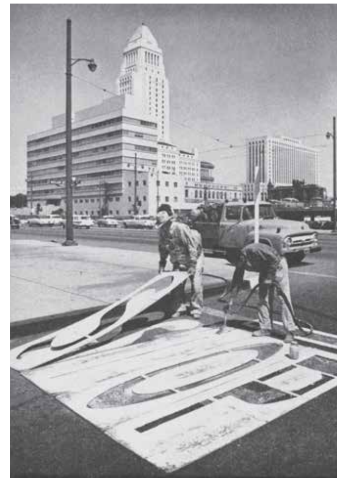
LEFT: Road marking with plywood stencils.
